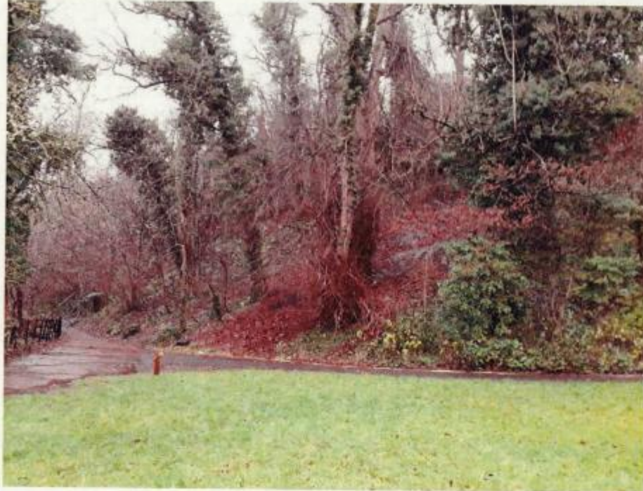
Figure 8b: View of slopes at chainage 170 m
